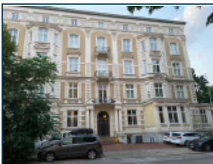
The family house now home to the Hamburg Waterways and Shipping Office
